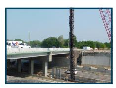
When the full single-point urban interchange (SPUI) is complete it will allow for opposing left turns to be made at the same time, compared to the previous diamond interchange that had two signals for the I-70 ramps. With only one set of traffic signals, more vehicles can make the turn and clear the interchange in one traffic signal cycle. SPUIs also allow for long, gradual turns giving larger vehicles like trucks, buses and recreational vehicles more room to navigate.
