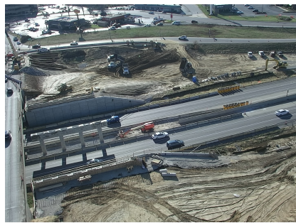
» Cave Springs Interchange in December 2022
