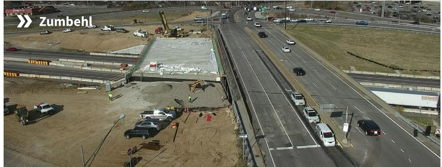
Girders were placed over I-70 at Zumbehl in late October and the bridge driving surface was poured in November. Also in November, crews built the substructure and bridge walls at Cave Springs.
